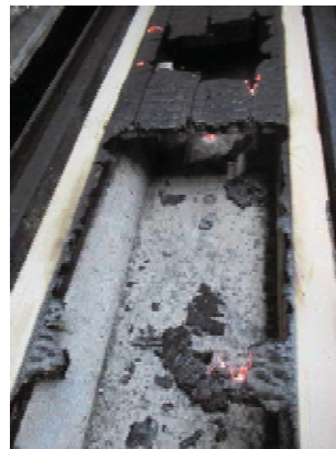
Small Pieces Falling/破片落下
